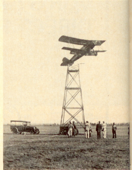
The Tanager climbing over the 35-foot barrier from a standing start 500 feet away—one of the requirements of the Guggenheim safety contest.
